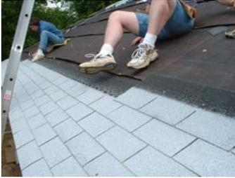
Shingle joints are "staggered" so that any upper shingle covers the joint between the sides of the shingle below. Thus, each shingle is sealed by another shingle. A thin ribbon of tar on the back of every shingle (seal tab) assures that the bottom of every shingle is securely bonded to the shingle below in case of wind. Proper nailing is so important that it is necessary to review the procedure each time Habitat volunteers install a roof.
